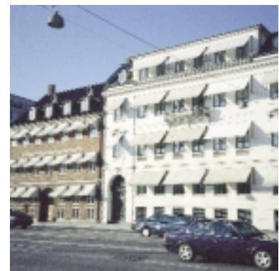
Retrofit: retractable fabric awnings (Source: J Goulding, ERG)
